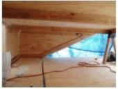
Andy wanted a very stiff cabin deck. He chose two layers of ½" ply sandwiching 1½" blue foam, stiffened by 2x4 framing. My only quibble is that I would've liked to see liquid polyurethane used to fill cracks and gaplets (rather than spray expansion foam, which struck me as hardening too quickly to achieve real penetration). In the worst case scenario, though, in twenty years he can zip the whole deck off, if necessary, and do it again in a matter of days.
